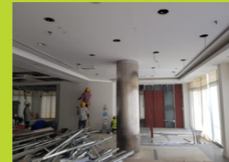
Before & After Demolishing
