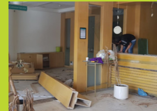
Before & After Demolishing
