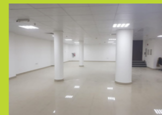
Tiling, Ceiling & Painting
